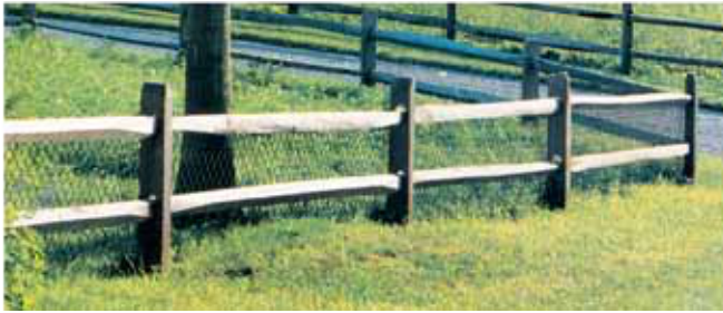
Coated wire mesh applied to split-rail fencing may be used for pet enclosures.
