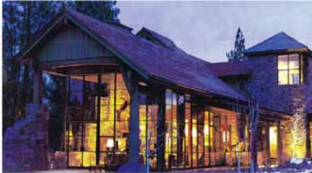
A modern interpretation of the Rustic Mountain House utilizes large areas of recessed glazing under projecting roof overhangs to connect interior spaces to the outdoors.
