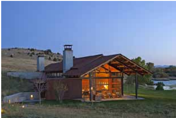
Buildings are to evoke the outdoor lifestyle of the region by including exterior living spaces.
