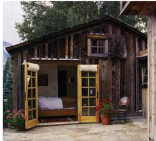
Traditional vertical wood siding on a Western Ranch house.
