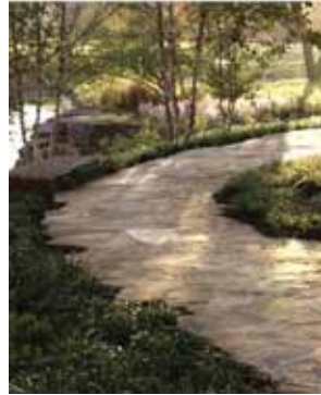
Native Montana flagstone set on a concrete base.
