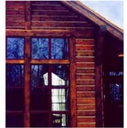
Horizontal timber siding (stacked timber wall)
